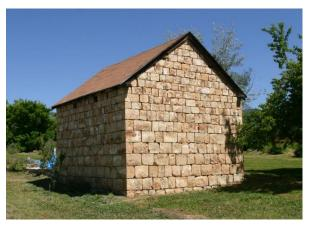
This stone building served as the town jail from 1874 to 1899. This small stone building is essentially a cabin type structure. The square plan has a three-opening, window/door/window façade. A single wooden lintel beam supports all three openings of the former jail.
