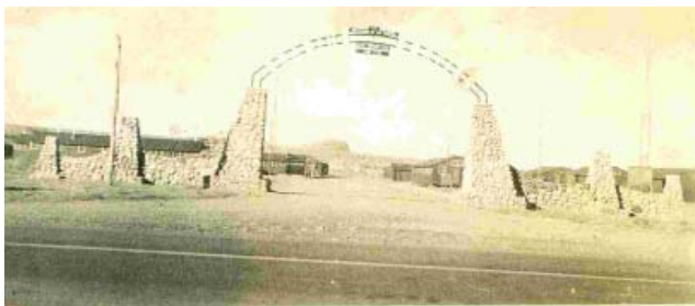
Entrance to the Civilian Conservation Service Camp, Dry Valley, Utah.
