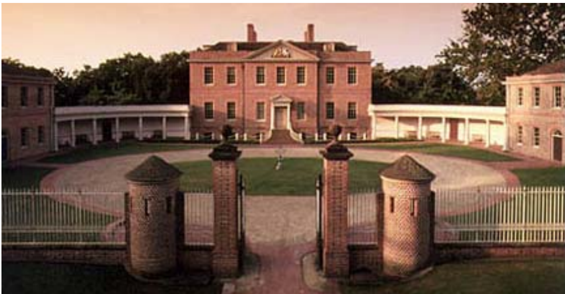
Tyron Palace, New Bern, NC, was home to the British Governor. The palace has been reconstructed and it available for tours. Taxes from the Colonists, including the Allreds, helped maintain this facility.
