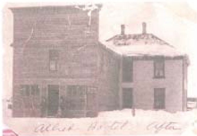
Allred Hotel and Store under construction in Afton, Wyoming.
