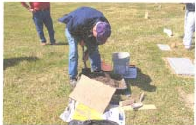
Franklin Allred prepared the cement for the stone setting.
